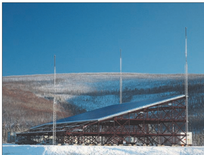
The first complete face of the AMISR system at Poker Flat in October 2006. Since each face of AMISR can function independently, when the system is completed it can be deployed in up to three separate locations at the same time. The first AMISR face is expected to remain at Poker Flat until at least 2010. Photo courtesy Craig Heinselmann.
