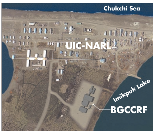
An aerial view showing the location of UIC-NARL and the five phases of the new Barrow Global Climate Change Research Facility (BGCCRF). Courtesy of LCMF LLC. Photograph © AEROMAP US.
